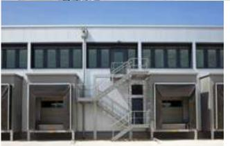
Anticorrosion protection of the steel parts was carried for reasons of industrial pollutants due to installation in the Industrial Area of Patras plus small distance from the sea.
