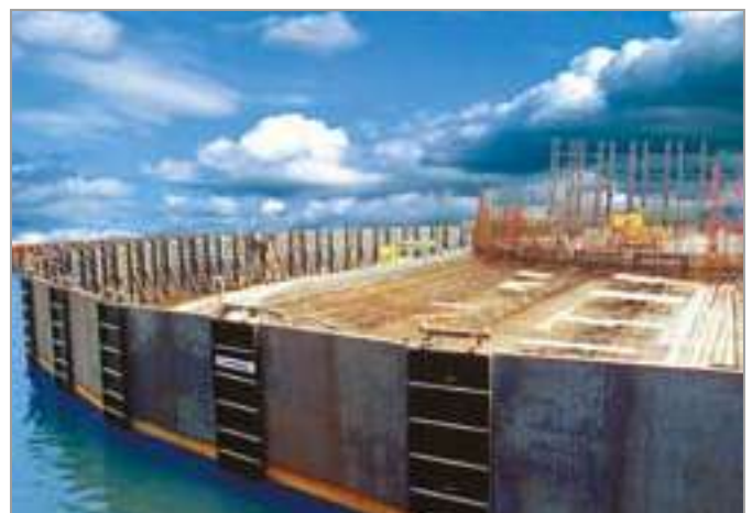
Steel retaining wall (Gefyra Joint Venture)
